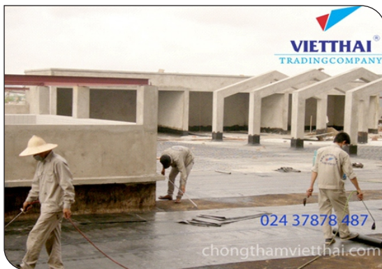
Construction of torched on membrane
